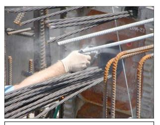
$MCI^{\circledast}$ -309 is applied as an aerosol suspension (dry fogging) into the casing surrounding the metal element to prevent corrosion.
